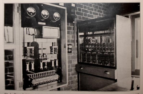
Fig. 4.—Power Switchboard (left) and Contactor Case (right) in upper part of Signal-Box. Batteries in lower part of Signal-Box.
